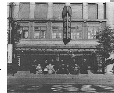
Headquarter at the foundation
